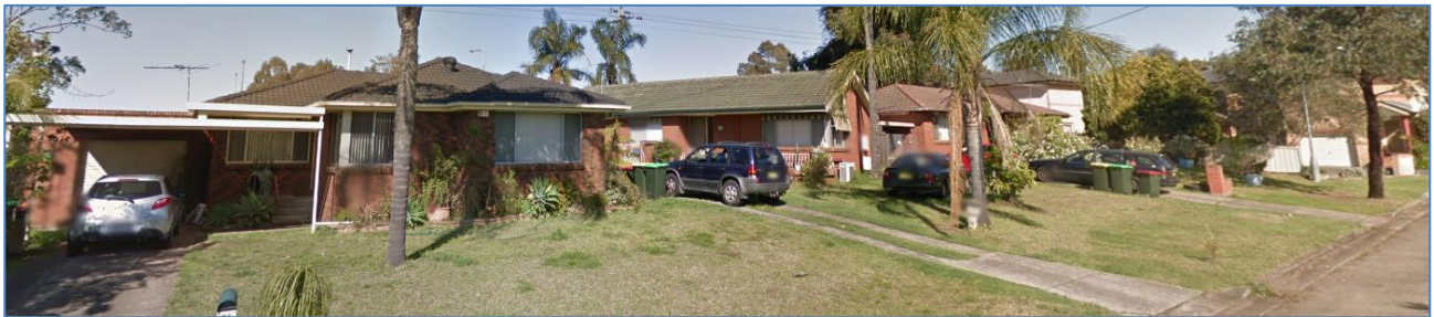
Figure 1.4 Properties to be demolished
